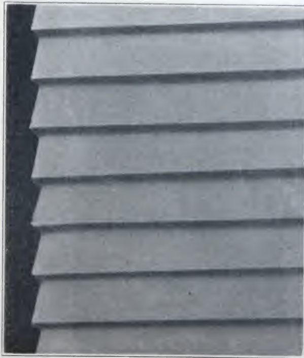
CYPRESS SIDING WITH MITERED CORNERS
